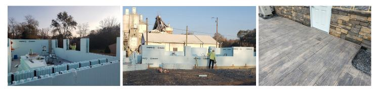
Choosing to use ICF decking (Insuldeck) to construct the roof added to the challenge. We opted to go with a concrete roof in order to accommodate future vertical expansion of the building.
