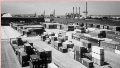
RCC's high strength stands up to heavy loads and special equipment at port and intermodal facilities
