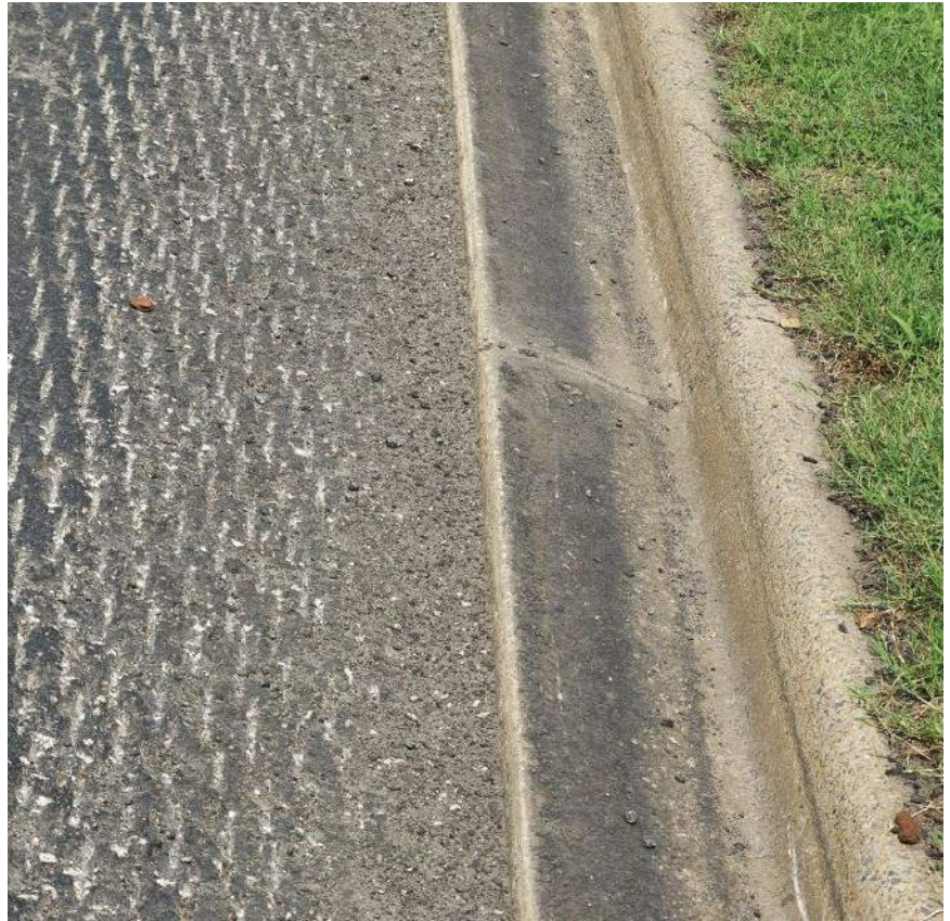
Existing pavement milled 2 inches below gutter.
