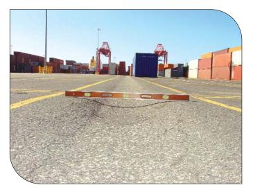
Rutting in asphalt pavement caused by channelized loading.
