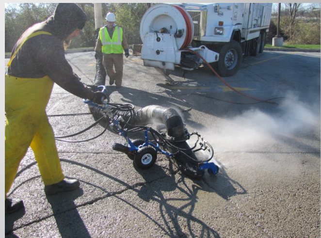
Cleaning pervious concrete
