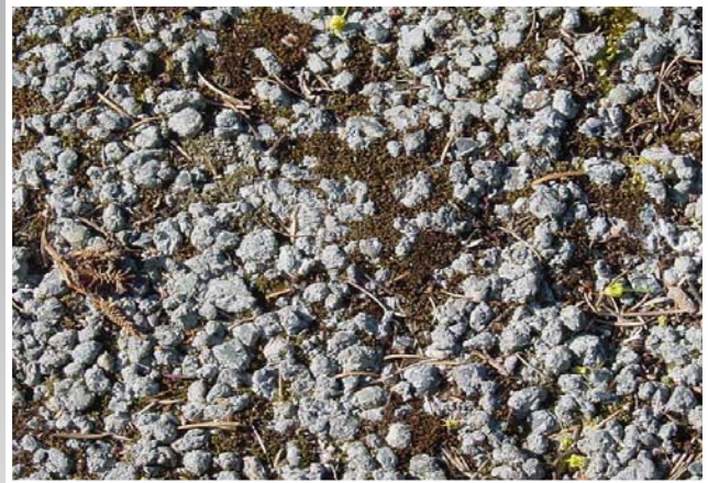
Pervious Concrete: Post-maintenance
