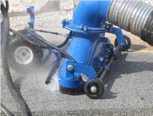
Cleaning pervious concrete
