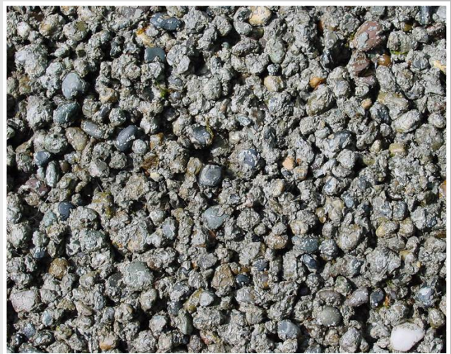
Pervious Concrete: Pre-maintenance
