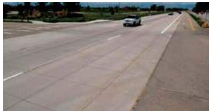
Figure 20. SH-119 in 2009 after 18 years of service (source: Ron Youngman, CO/WY chapter, ACPA)
