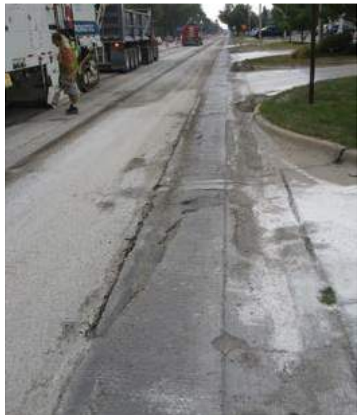
Figure 119. Typical concrete pavement milling operation (source: Dan DeGraaf, Michigan Concrete Paving Association)
