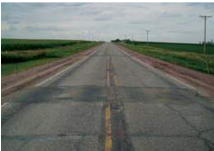
Figure 39. Composite pavement prior to unbonded concrete overlay
