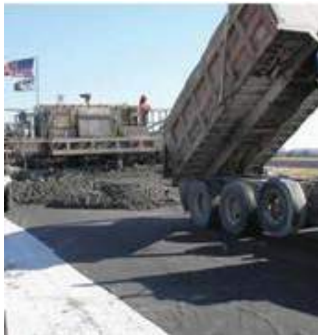
Figure 112. Paving on top of nonwoven geotextile materials
