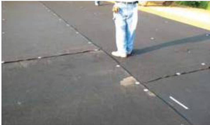
Figure 110. Overlap of nonwoven geotextile material section
