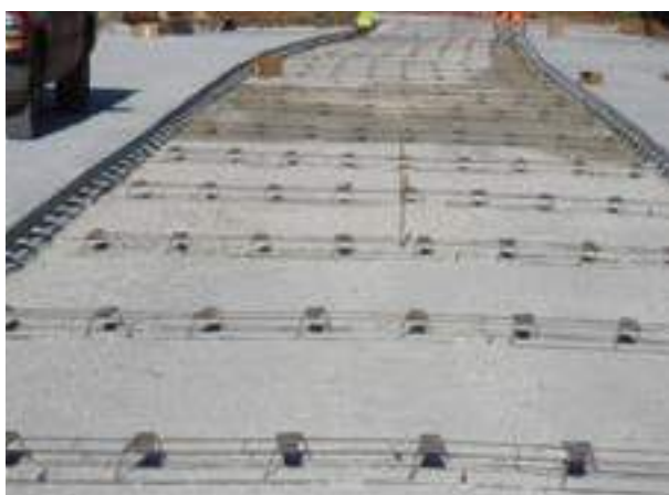
Figure 54. Tapered plate dowel baskets in transverse contraction joints and football-shaped plate dowels for slipformed longitudinal construction joints
