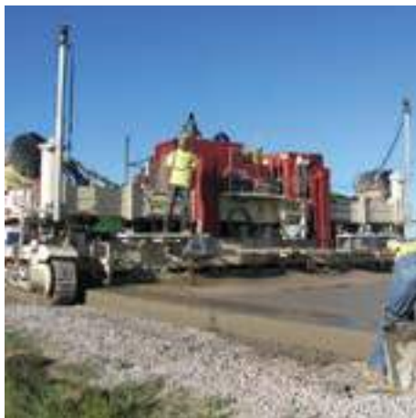
Figure 140. System 2 paving machine
