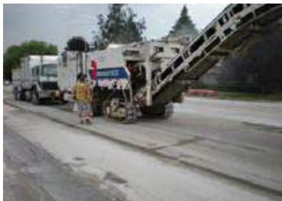
Figure 3. Milling concrete (left) and milled surface (right)
