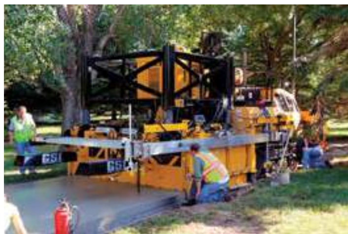
Figure 101. Zero clearance stringless paver (source: GOMACO)
