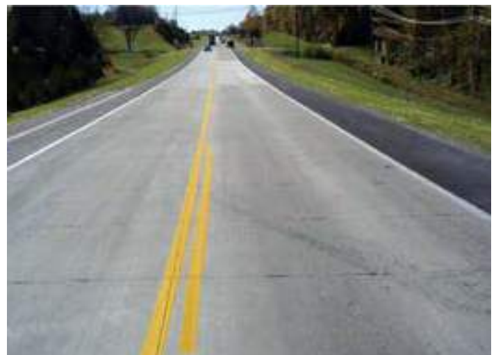
Figure 45. Route D35 5-inch unbonded overlay (source: Todd LaTorella, MO/KS Chapter, ACPA)
