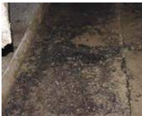
Figure 53. Asphalt stripping of interlayer (source: Dan DeGraaf, Michigan Concrete Paving Association)
