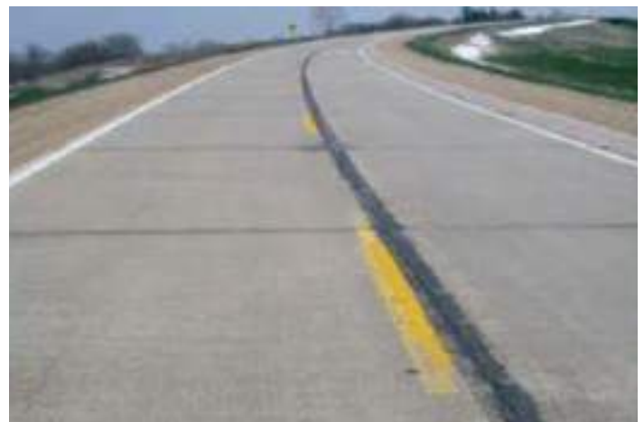
Figure 29. Three-inch concrete bonded overlay (photo dated 2013) (source: Todd Hanson, Iowa DOT)
