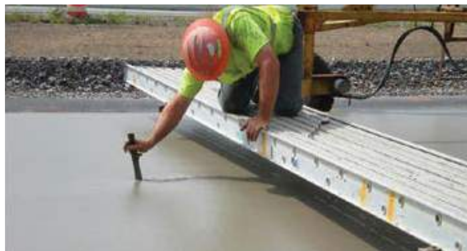
Figure 115. Manually verifying dowel placement
