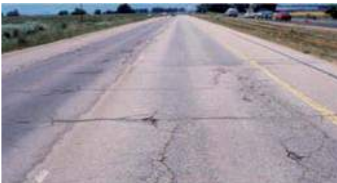
Figure 19. SH-119 in 1991 prior to placement of an bonded concrete overlay (source: Ron Youngman, CO/WY chapter, ACPA)
