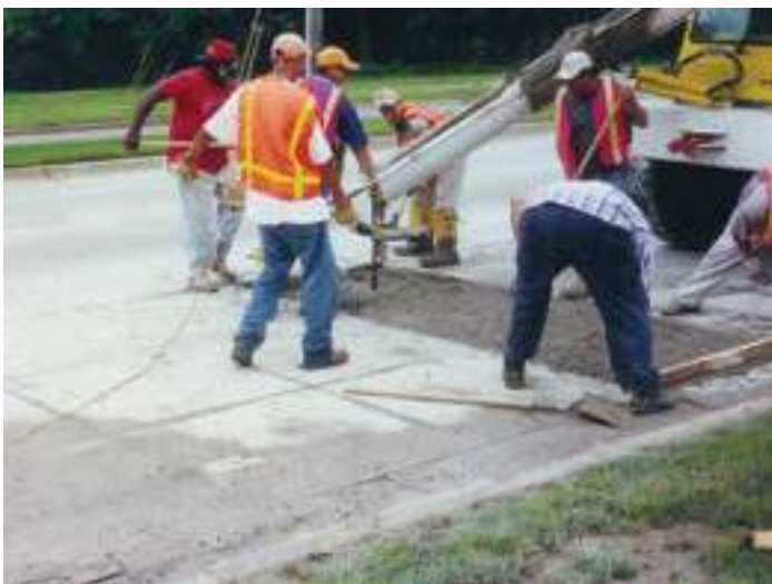
Figure 117. Finish and cure of concrete overlay repair (source: Dan DeGraaf, Michigan Concrete Paving Association)
