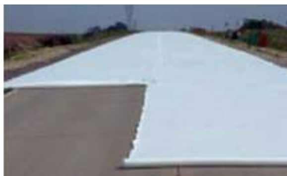
Figure 51. White geotextile fabric separation layer (source: Larry Engbrecht, South Dakota ACPA)
