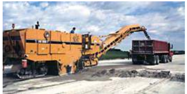
Figure 118. Typical concrete pavement milling operation (source: Randell Riley, Illinois chapter, ACPA)
