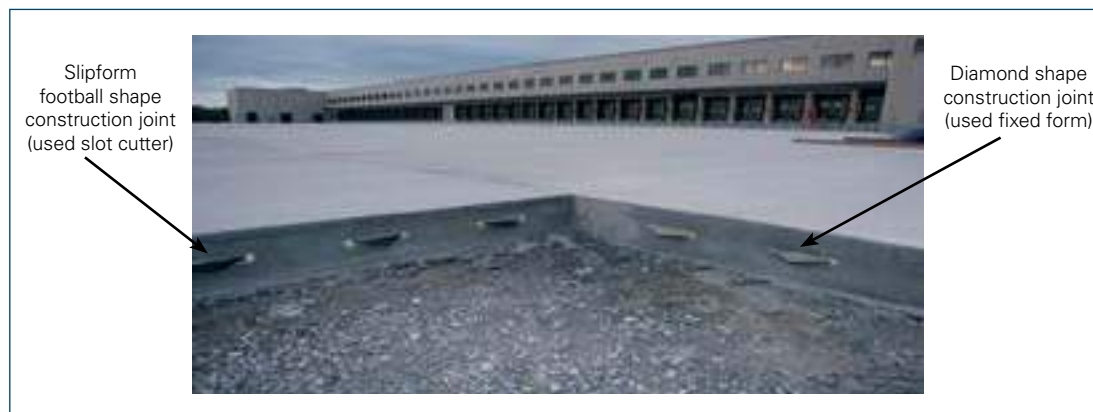
Figure 65. Diamond-shaped plate dowels in fixed-formed construction joints (right side) and football-shaped dowels by slipforms
