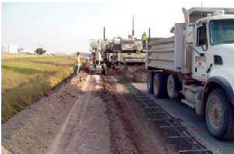
Figure 82. View of tiebars for concrete overlay widening unit
