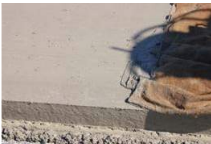
Figure 125. Finished concrete overlay with synthetic fibers
