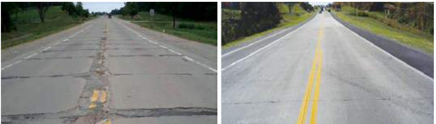
Figure 1. Typical concrete overlay (before [left] and after concrete overlay placement)
