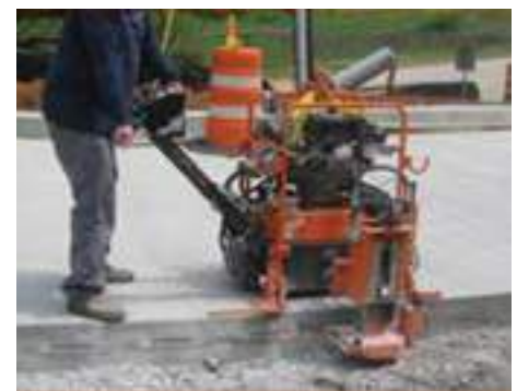
Figure 69. Slots being cut to accept the football-shaped plate dowels (source: Nigel Parks, PNA Construction Technology)
