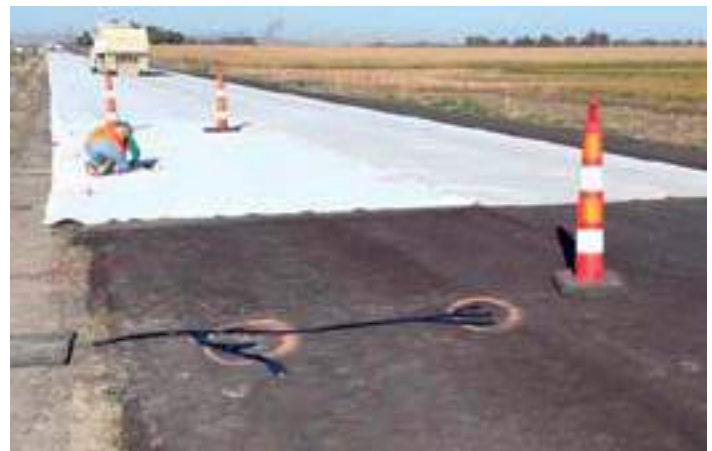
Figure 93. Light-colored geotextile fabric used as a separation layer for an unbonded overlay
