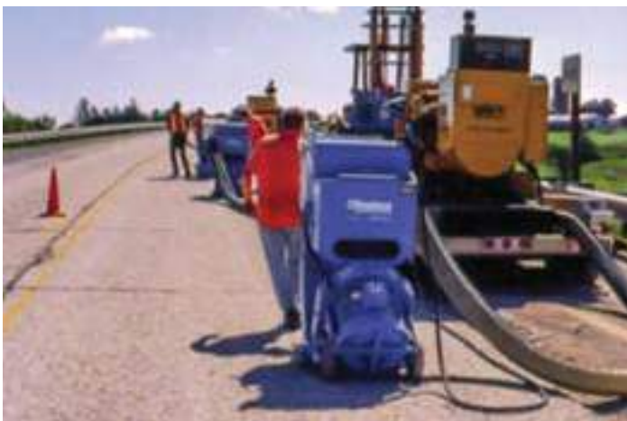
Figure 28. Photo of concrete pavement with shotblast surface prior to concrete overlay in 1994 (source: Todd Hanson, Iowa DOT)
