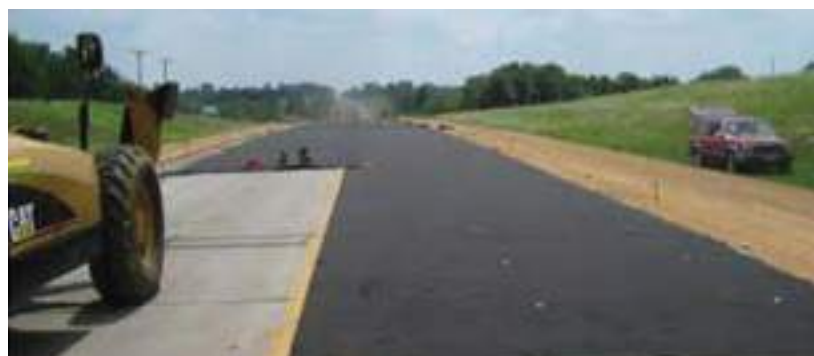
Figure 50. Geotextile fabric separation layer (source: Missouri DOT)
