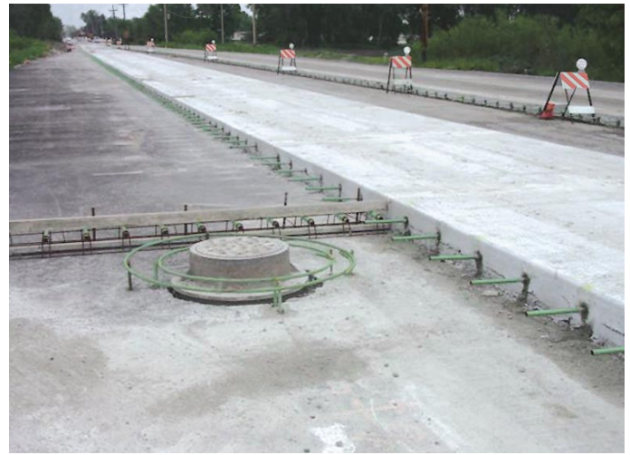
Figure 11. Dowels, tiebars and utility fixtures in position for fixed-form paving.
