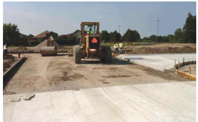
Figure 9. Compacting subbase.
