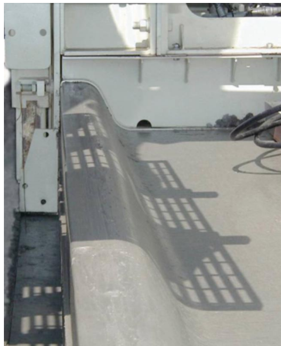
Figure 13. Slipform pavement with integral curb.
