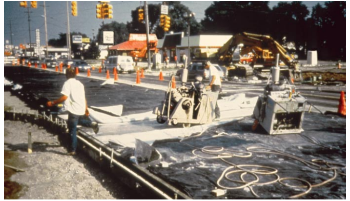
Figure 14. Curing blankets moved aside for sawing fast-track concrete.
