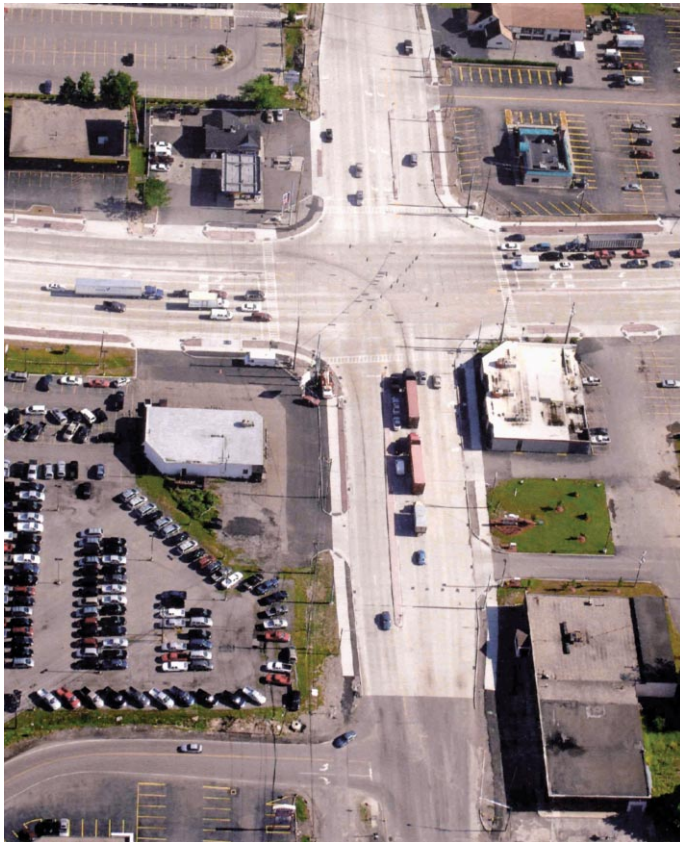
An intersection reconstructed with concrete.
