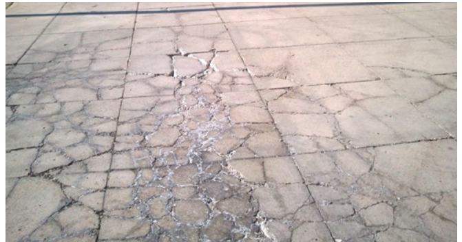
Figure 10. Concrete overlay failure resulting from inadequate information about support conditions
