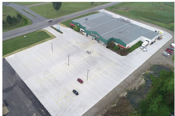
Figure 57. Completed concrete overlay on the parking lot of Super Ron's Food Center in Pulaski, Wisconsin (2021)
