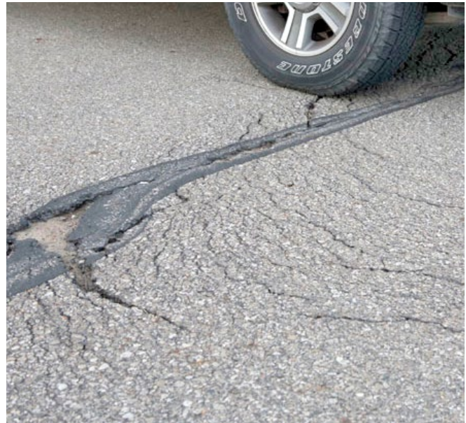
Figure A-16. Low- to medium-severity shoving
