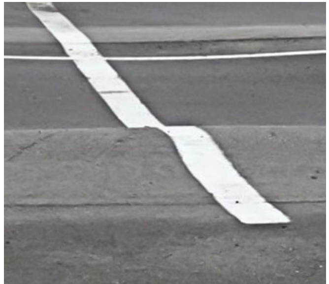
Figure A-15. High-severity rutting
