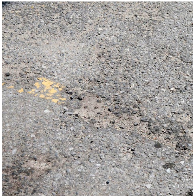
Figure A-8. Low- to medium-severity raveling
