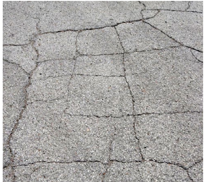
Figure A-4. Low- to medium-severity block cracking
