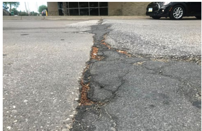
Figure A-17. High-severity shoving
