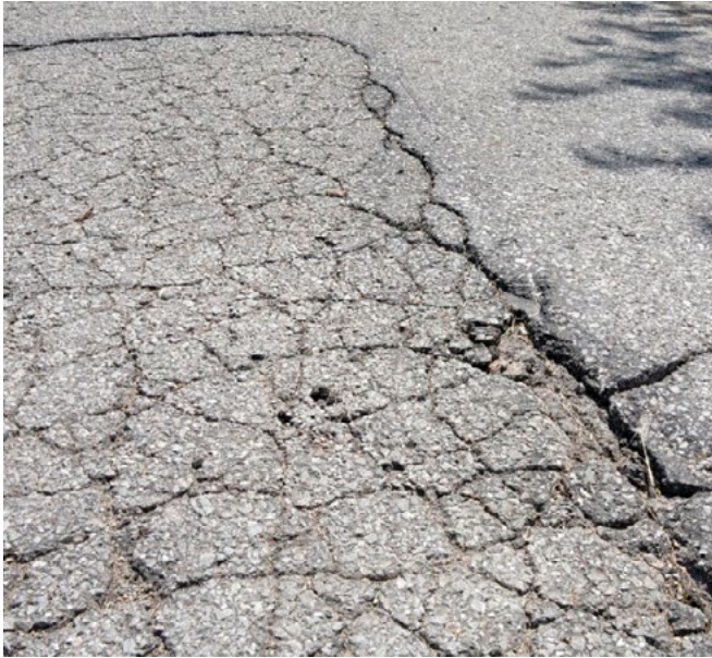
Figure A-3. High-severity alligator cracking
