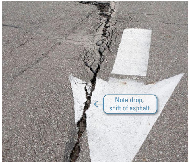
Figure A-11. High-severity thermal cracking
