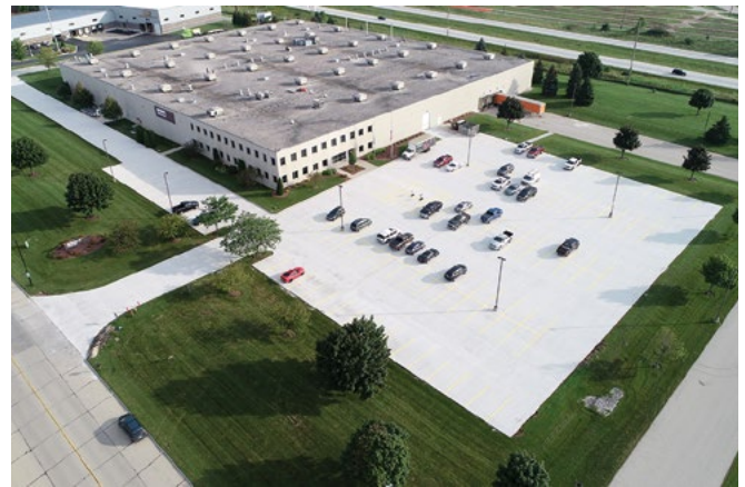
Figure 59. Completed concrete overlay on the parking lot of the Parker-Hannifin facility in Manitowoc, Wisconsin (2021)
