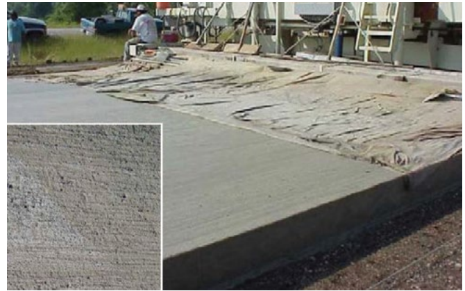
Figure 44. Burlap drag texturing and the resulting texture
