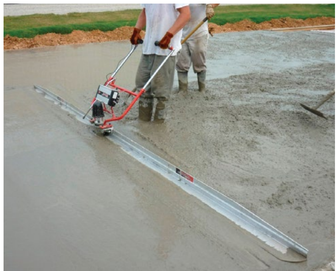
Figure 33. Handheld vibrating screed
