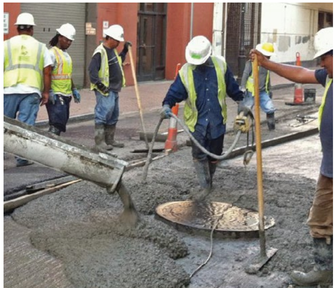
Figure 32. Concrete vibrator
