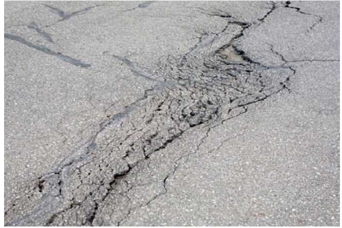
Figure A-6. Low- to medium-severity pothole
