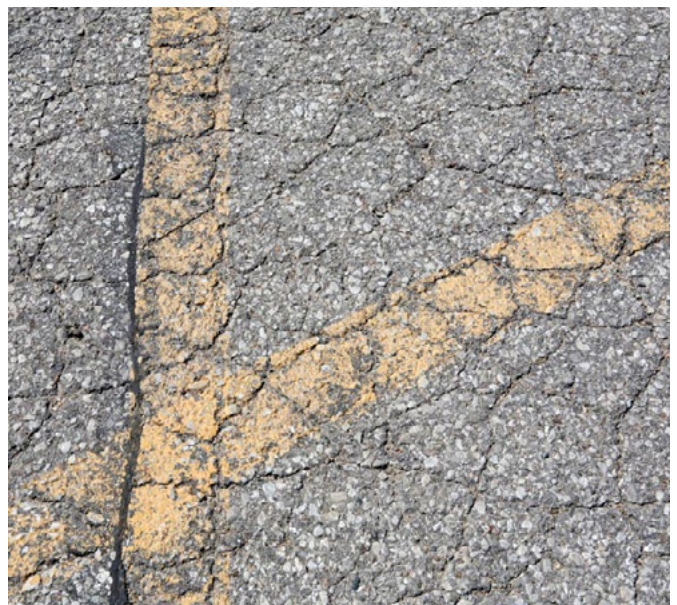
Figure A-2. Low- to medium-severity alligator cracking
