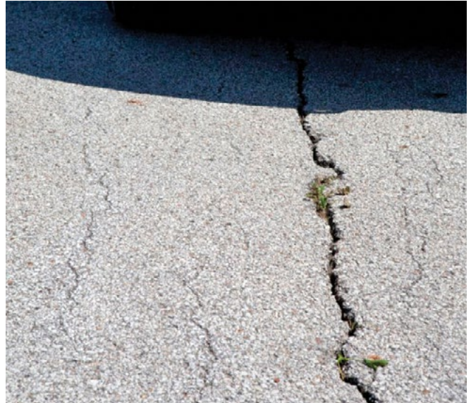
Figure A-10. Low- to medium-severity thermal cracking
