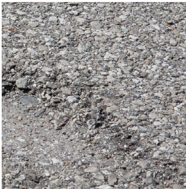
Figure A-9. High-severity raveling
