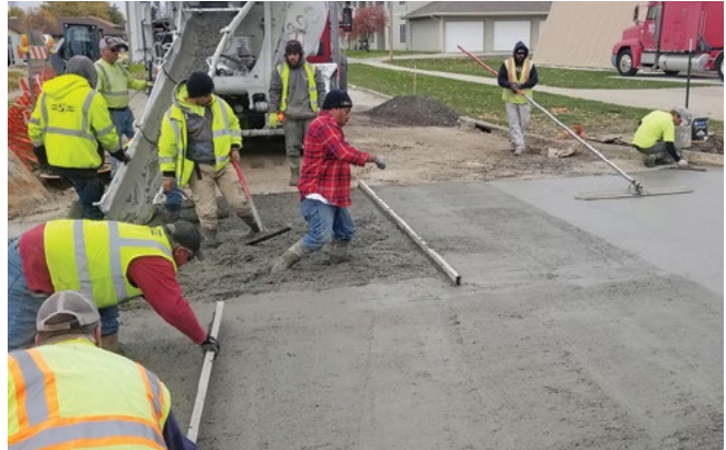
Figure 31. Striking off with hand/wet screed
