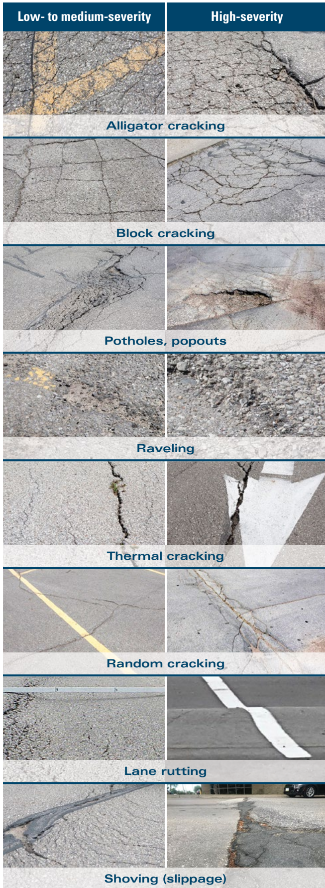
Figure A-1. Thumbnails of asphalt pavement distresses
