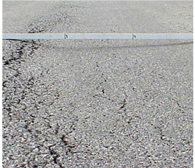
Figure A-14. Low- to medium-severity rutting
