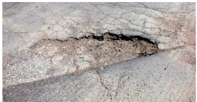
Figure A-7. High-severity pothole
