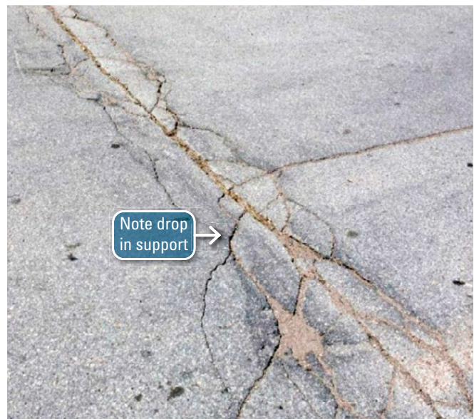
Figure A-13. High-severity random cracking
