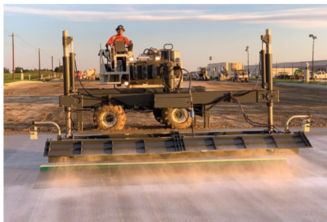
Michael Hoeft, K & M Concrete Construction, Inc., used with permission
