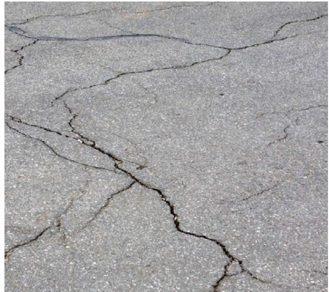
Figure A-12. Low- to medium-severity random cracking
